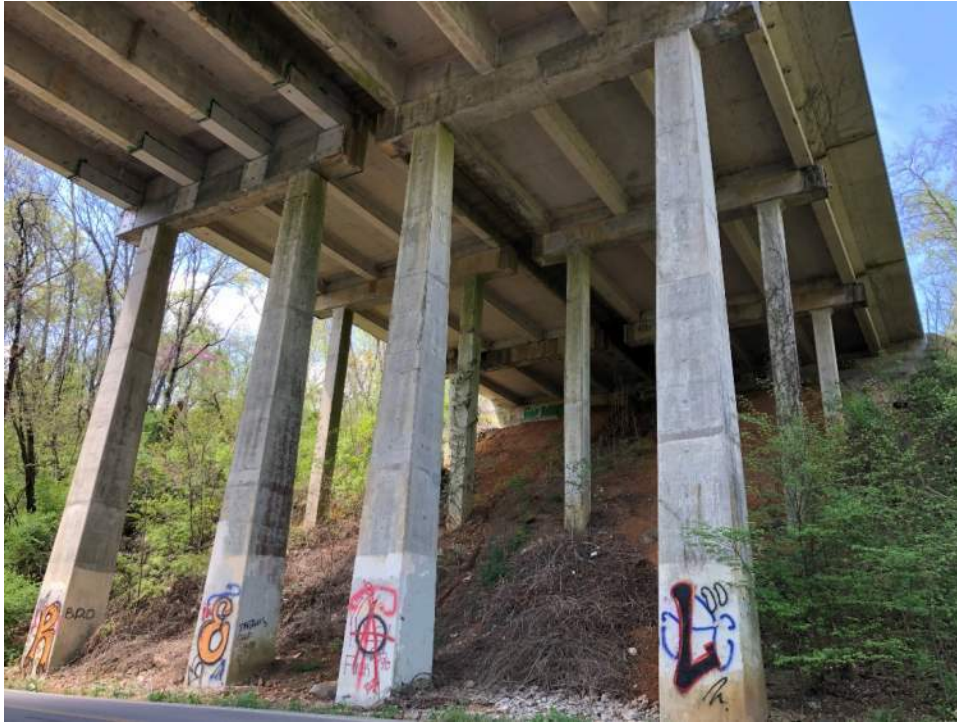
West bridge abutment (inlet side) wall, piers and beams
