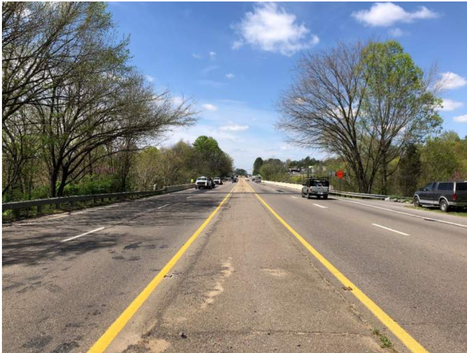
Looking west along east bridge approach
