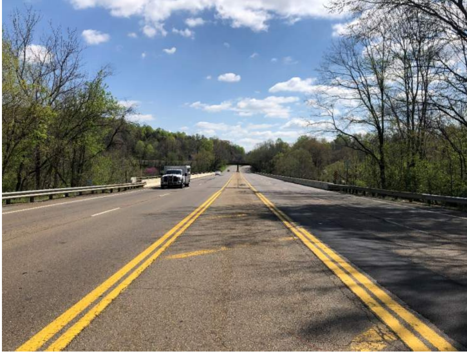
Looking east along west bridge approach
