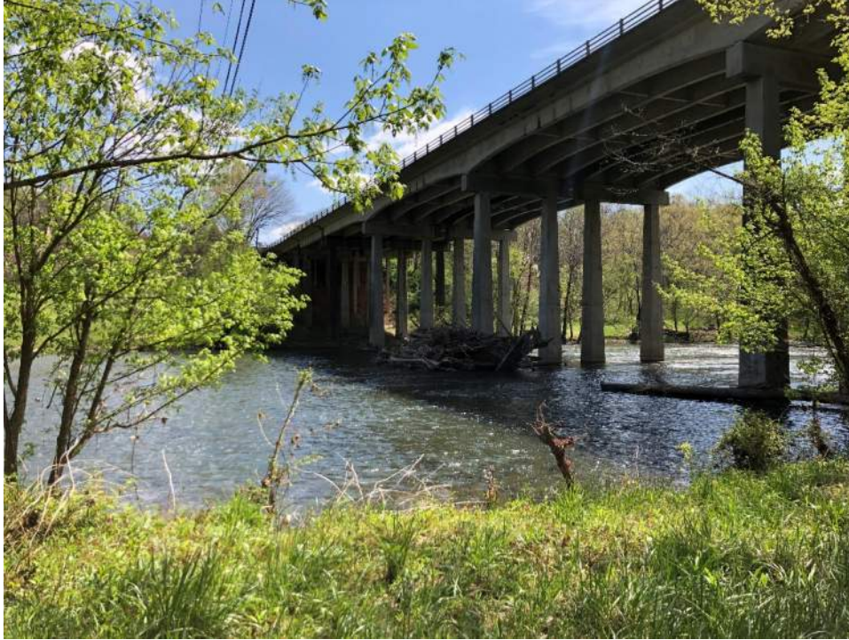
Looking southeast at bridge inlet
