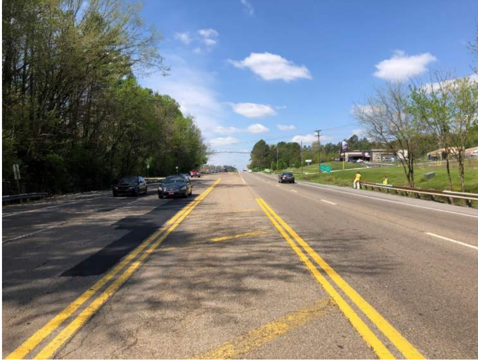
From bridge looking west along roadway
