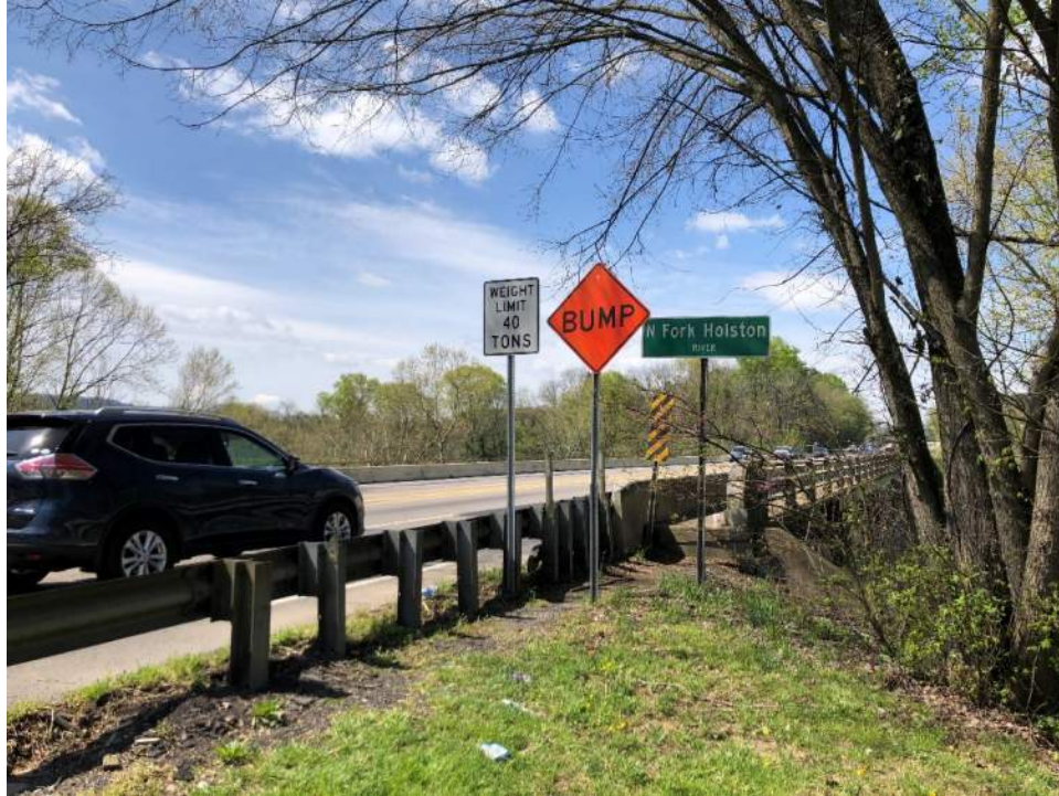
Weight limit sign before beginning of bridge on east approach
