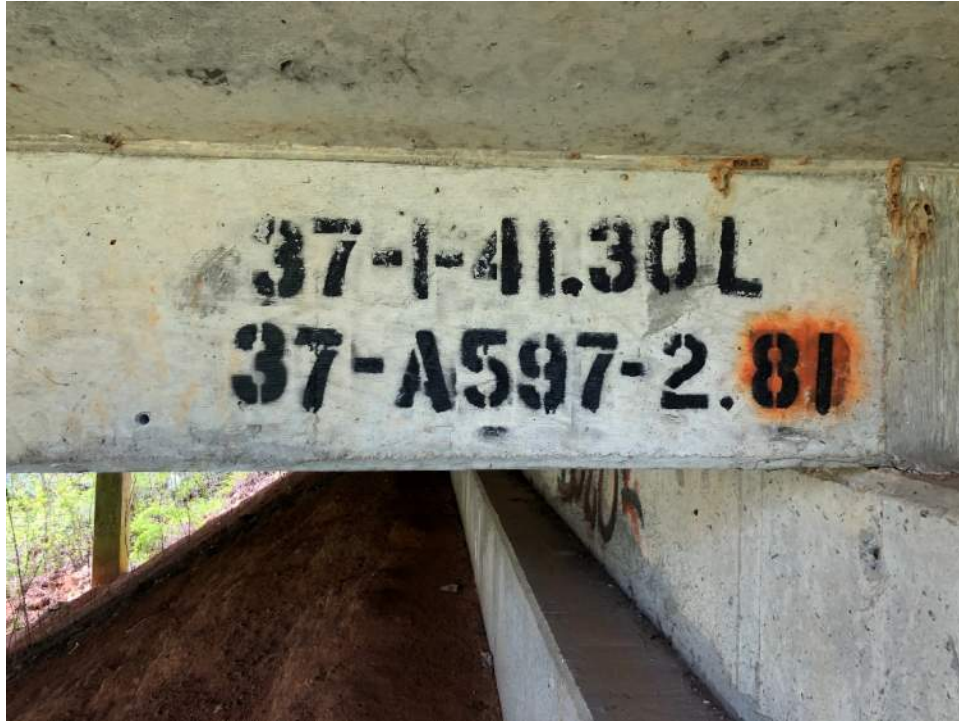
Bridge ID stamped on beam near west abutment wall
