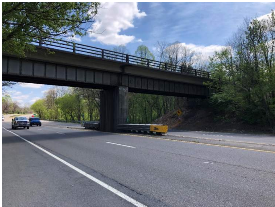
Railroad bridge (owned by CSX) on east bridge approach
