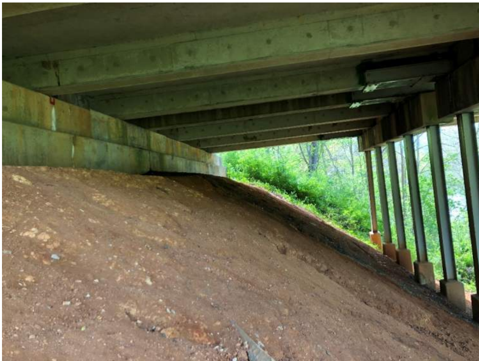
East bridge abutment (inlet side) wall, piers and beams
