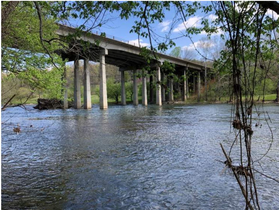
Looking northwest at bridge outlet
