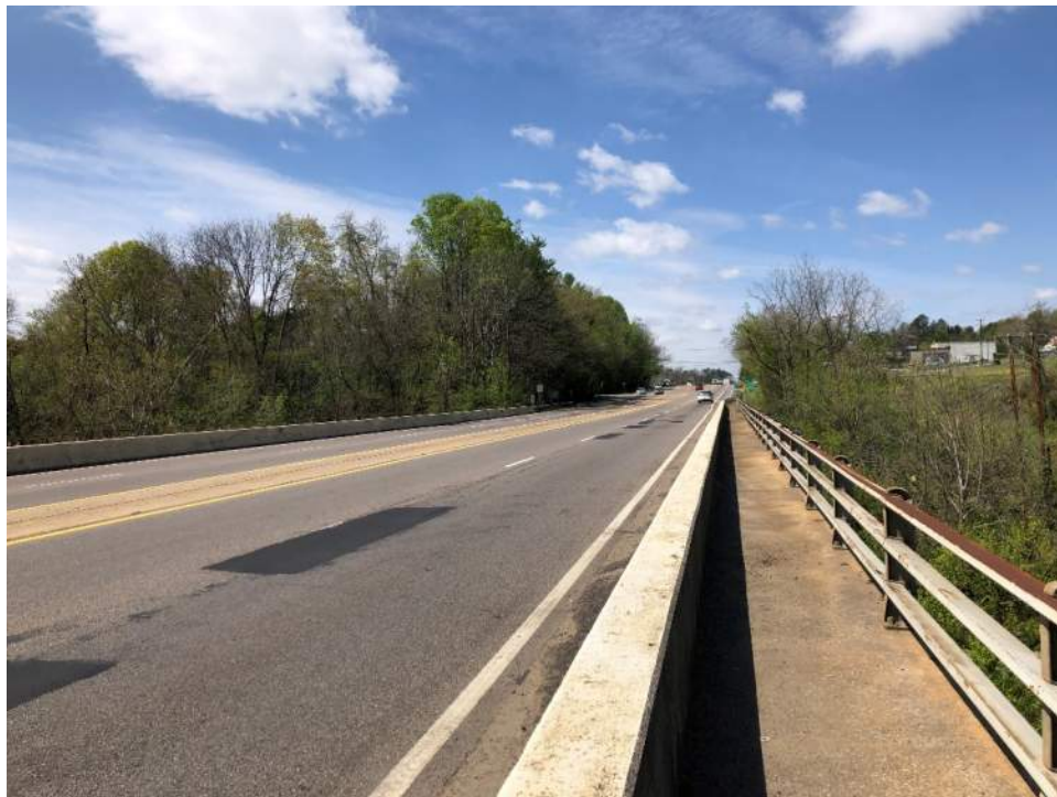
Concrete and steel rail system on bridge
