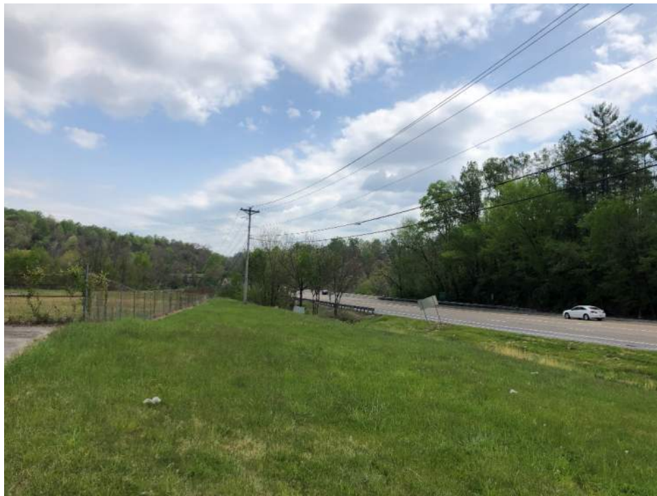
Utility lines north of bridge
